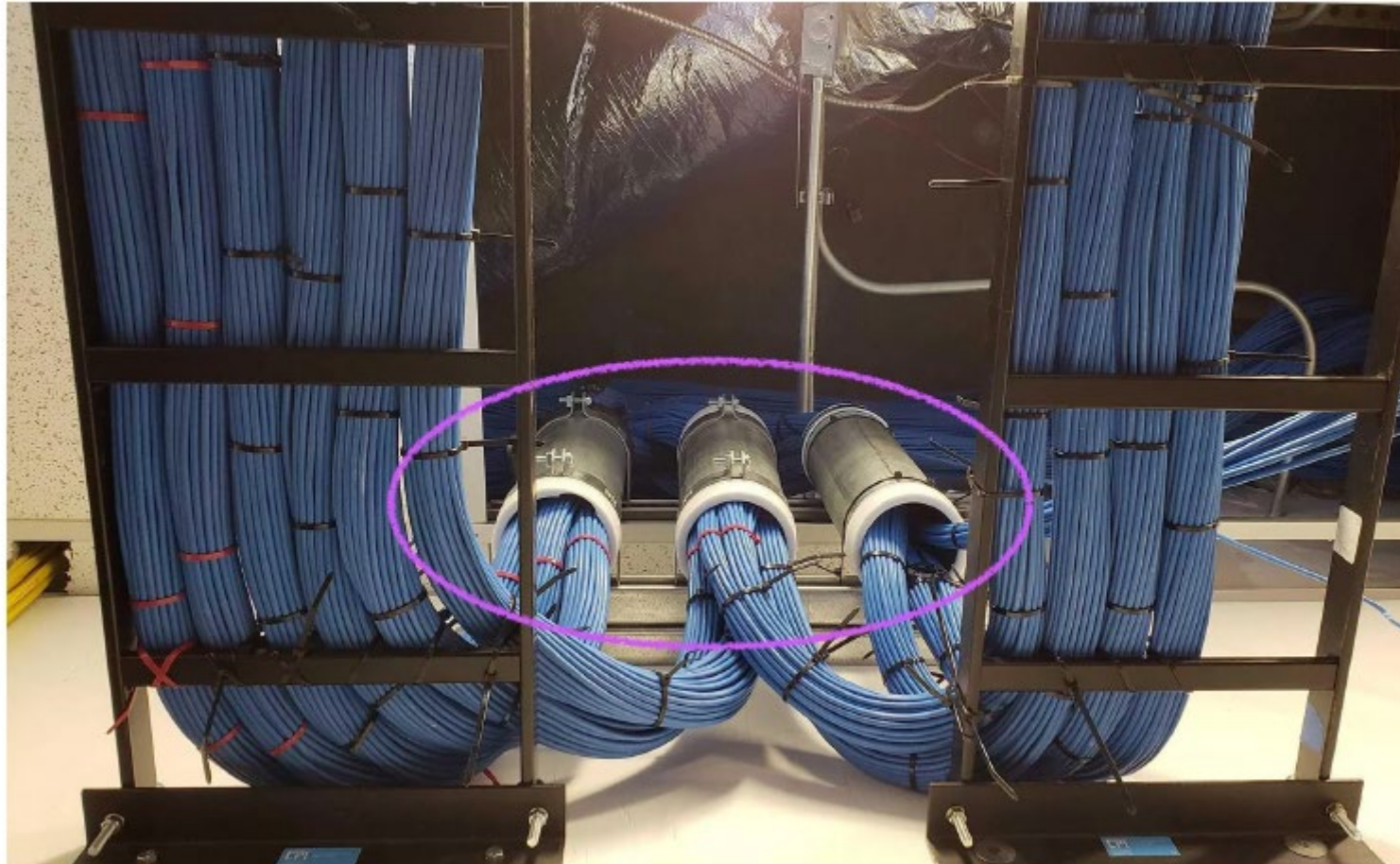
Chase pipe/conduit sleeve example
